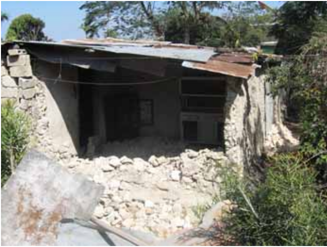
Figure 17 Home with Metal Roof
