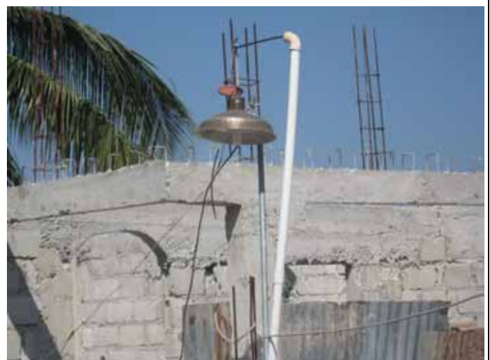
Figure 8 Beam with rebar to connect to floor slab (house under construction)
