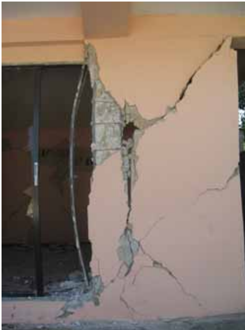
Figure 11 Building Column Reinforcement
