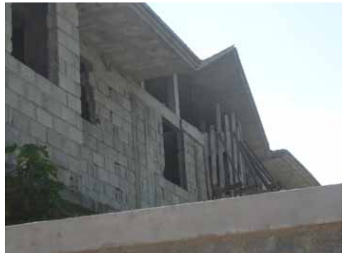
Figure 16 Interior Wall Reinforcement (house under construction)
