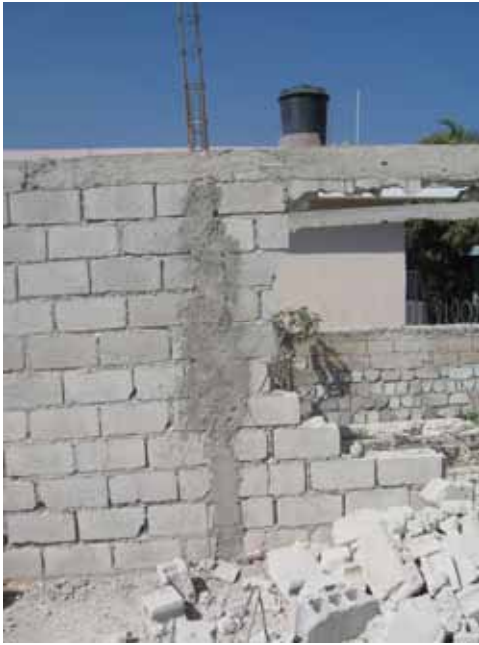
Figure 13 Interior Wall Reinforcement
