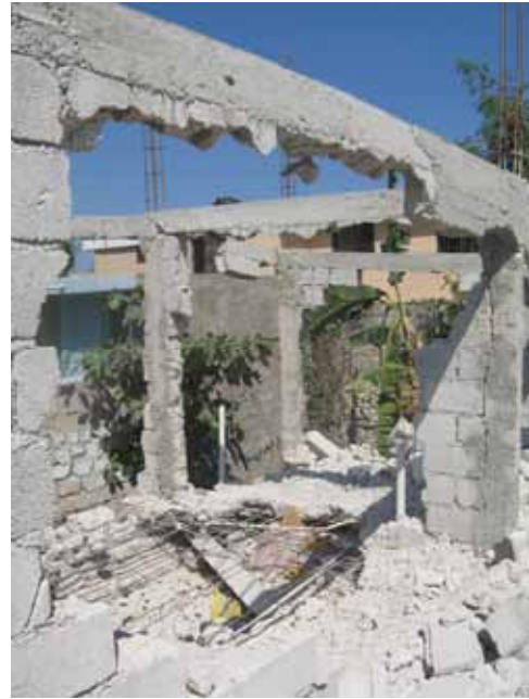
Figure 14 Interior Wall Reinforcement
