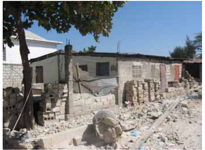
Figure 18 Home with Metal Roof
