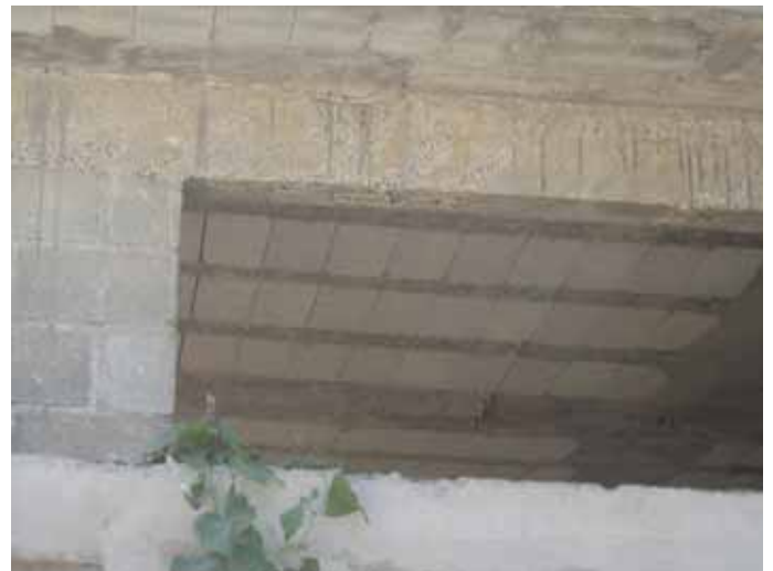
Figure 20 Concrete block slab
