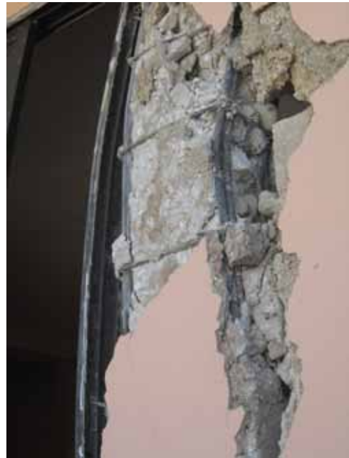
Figure 12 Building Column Reinforcement
