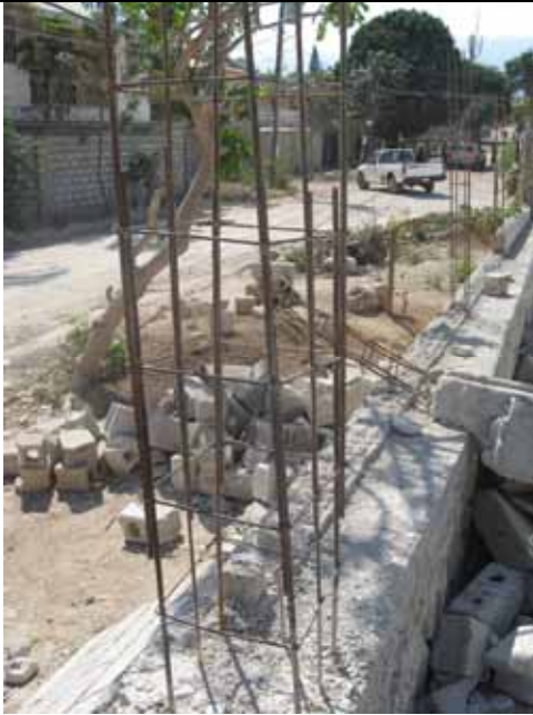
Figure 9 Building Column Reinforcement
