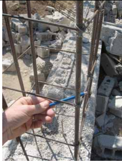
Figure 10 Building Column Reinforcement
