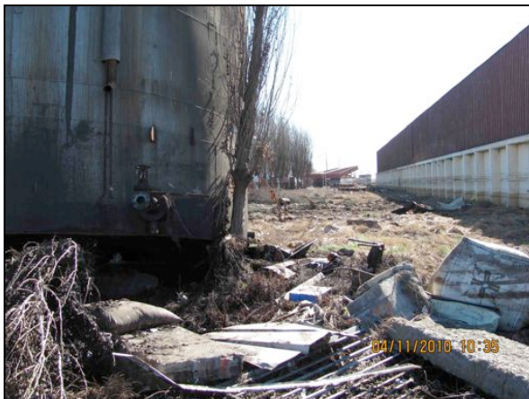
This fish oil tank was moved 300 m by the tsunami
