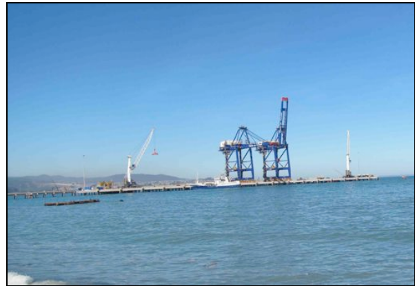
Pier #2, a base isolated pier-the part of the pier where the cranes are located did not have any damage
