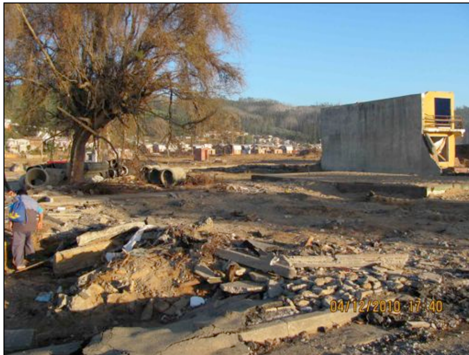
Dichato Tsunami damage
