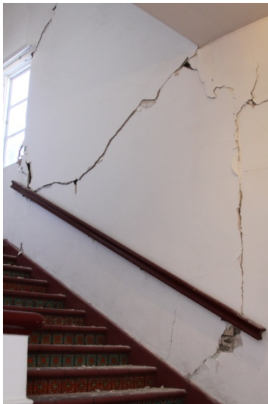
Figure 8. Typical interior damage of the Hotel de Anza in Calexico (images courtesy of professional photographer Joseph Llausas - taken April 6, 2010).
