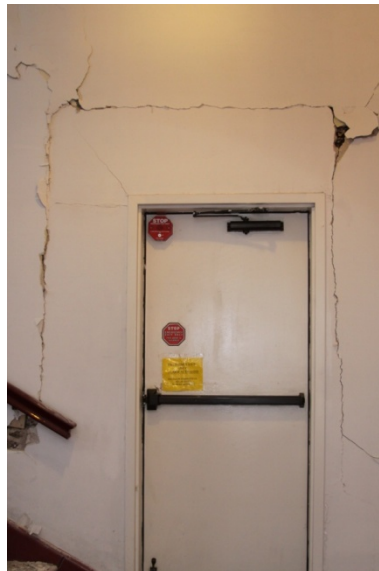
Figure 8. Typical interior damage of the Hotel de Anza in Calexico (images courtesy of professional photographer Joseph Llausas - taken April 6, 2010).
