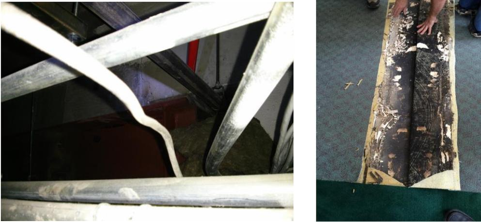
Figure 2: Precast beam and diaphragm connection damage at one location
