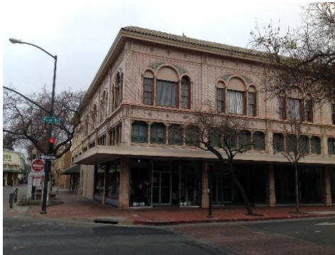
Figure 1 – Pre-Quake, Southwest corner
