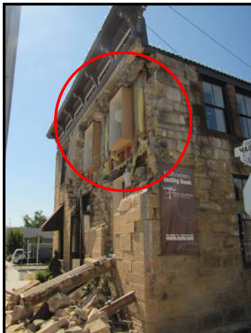
Damaged 1875-vintage stone masonry building in Napa. Note wall anchorage (through bolts with steel plates) in the close-up photo
