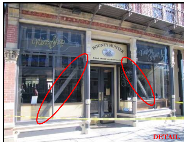
Retrofitted URM building that survived the earthquake. Upgrades included wall anchors and a steel braced frame at storefront.
