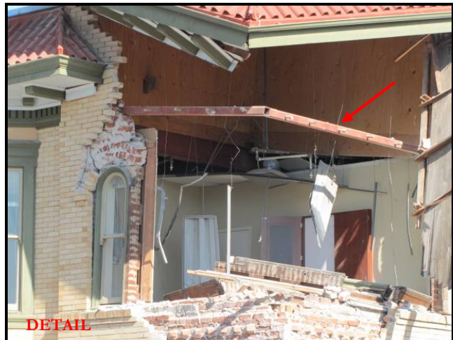
This three-story structure includes an unreinforced masonry façade, a portion of which collapsed onto the sidewalk below. The close-up photo shows remaining wall anchorage connections below the roofline.
