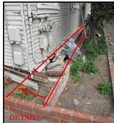
Residential wood-framed structures that predate modern seismic design consideration can shift from their foundations when short wood-framed walls are present surrounding the crawl space below the main floor. These common failures can lead to a fire-following-earthquake hazard from severed natural gas piping and nearby electrical components. Correcting this condition involves installation of plywood sheathing with floor and foundation connections.
